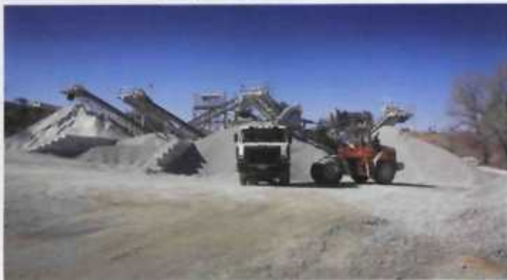
An AfriSam aggregate operation.
