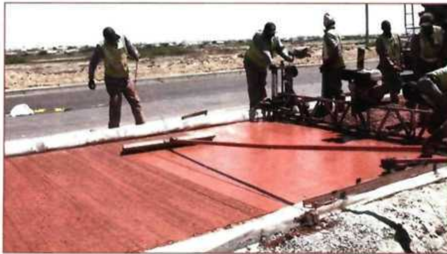
Work in progress on the Cape Town BRT bus lanes.
