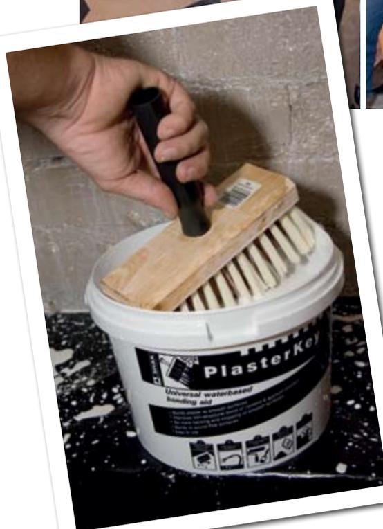
**Step 1** Clean your surface facebrick of any dust, dirt and mould, and patch up any holes or nasty imperfections. Coat the walls with plaster key – this will ensure the cement mixture bonds properly with the wall and won't crack or chip over time.
