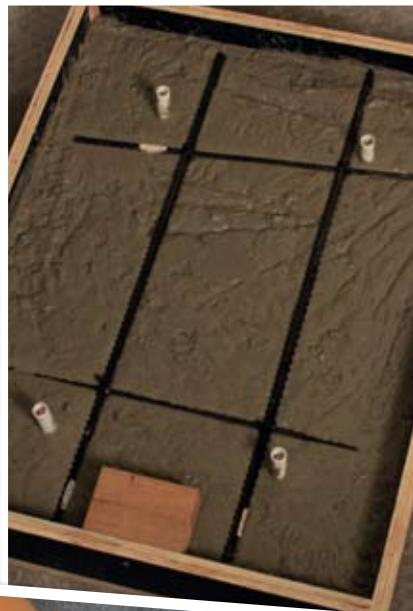
**Step 1** Start by making two moulds. Using black-faced shutterply board, cut four lengths to determine what thickness your slab needs to be (height, width and thickness all depend on your personal preference). Mix your concrete according to the recommended ratio. Don't use glue when assembling the mould, as you will need to remove it from the slab. Line the corners with wood filler for a smooth, round edge.
