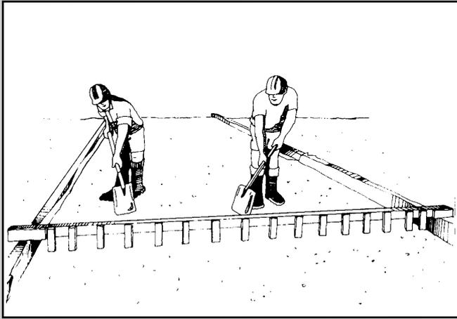
**Figure 3:** Trimming the excavation using a scratch template
